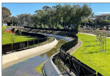
2 Glenside Detention Basin-Channel
