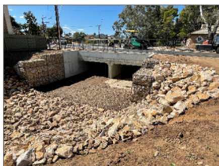
4 LBHC Daly Street Bridge
